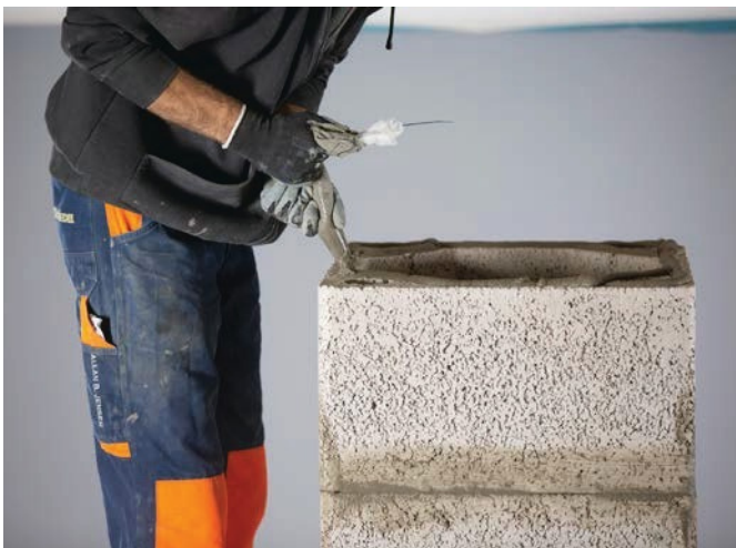
Apply jointing adhesive and install the next two chimney blocks, apply adhesive at every joint.
