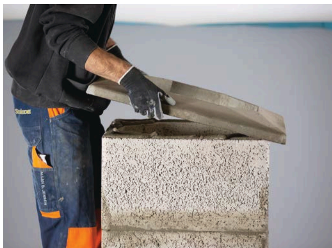
If the Top Cap is purchased, then apply a layer of jointing adhesive to the top of the final block and then press the Top Cap into place ensuring that it is level and wiping off any excess adhesive.
