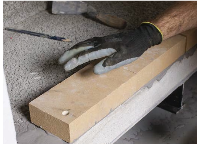
Bed the firebricks on to a 3mm layer of firebrick mortar. Use the tables on the previous page as a guide.
