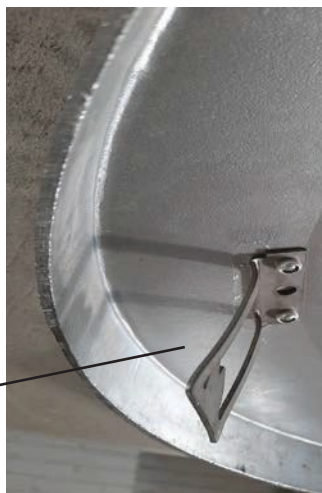
Bend the steel prongs out so the Rain Cap is a tight push fit into the concrete Top Cap.
