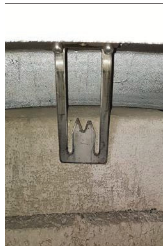
Bend the steel prongs out so the Rain Cap is a tight push fit into the concrete Top Cap.
