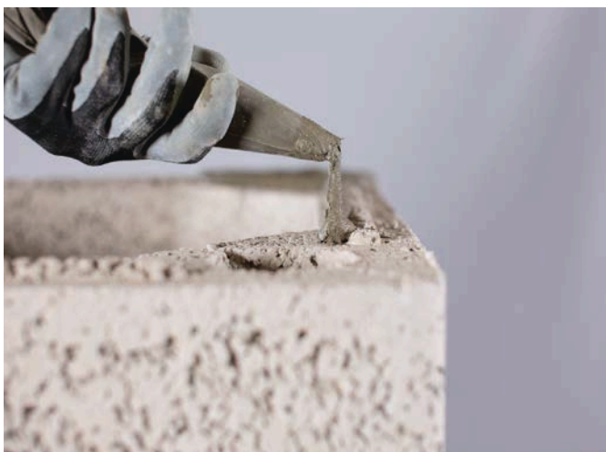
If extra Chimney Blocks are purchased, simply repeat the steps shown on p.4, applying a layer of jointing adhesive between each block and pressing the next block firmly into place. Ensure the top is level and clean off any excess adhesive.
