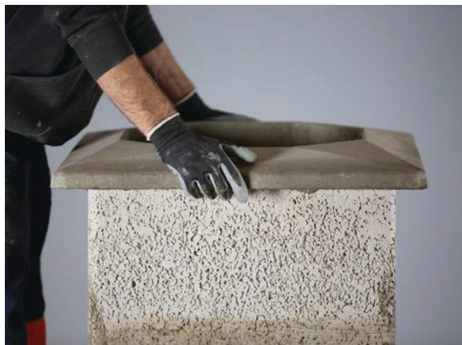
Apply jointing adhesive and install the optional Top Cap (if purchased).
