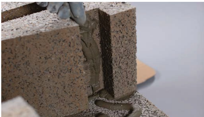
Press one side block into place and apply jointing adhesive into the slot as shown.
