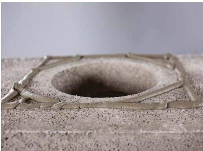
Spread jointing adhesive in the shape of the chimney block.
