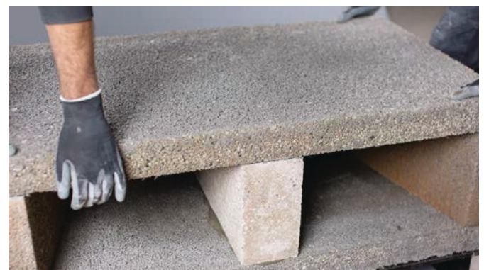
Press the base plate of the firechest down on to the log storage. Keep checking all is level and remove any excess jointing adhesive.
